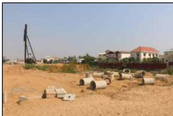
Construction near the International School of Phnom Penh (ISPP)
