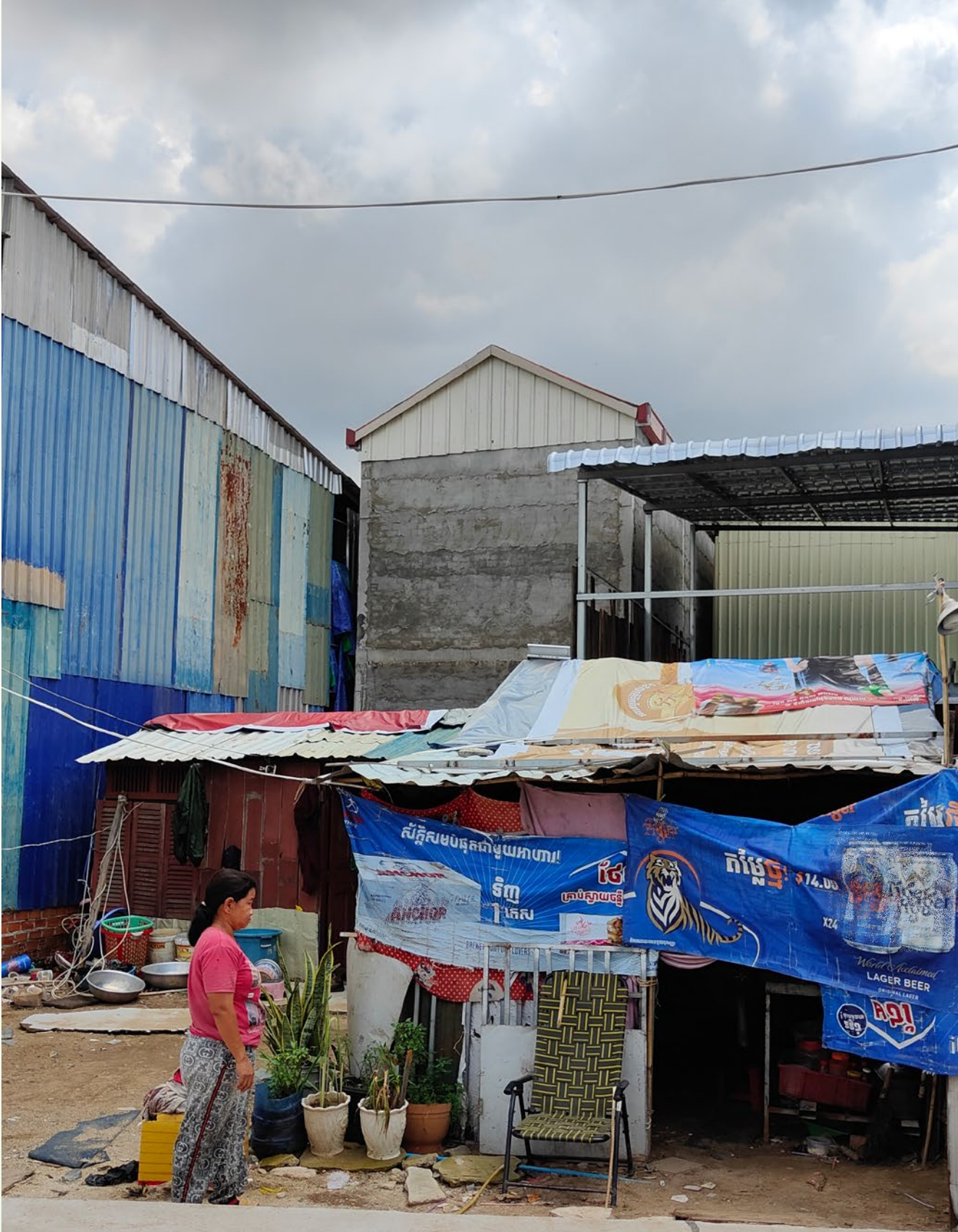
Picture 8: House condition at Champuh Ka'ek used old materials remain from previous location, 2024
