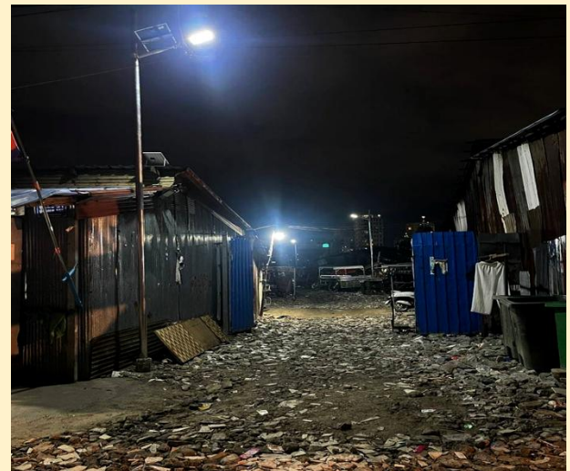
Picture of Solar Street light was Installed
